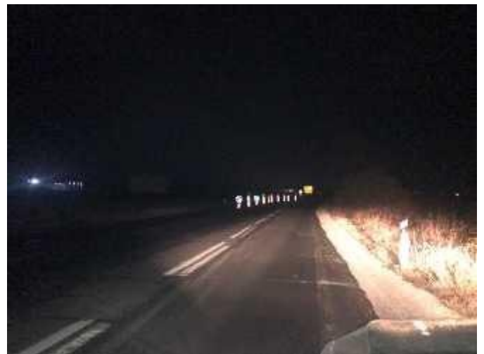
Fig. 4. Insufficient signaling construction site, section Prilep – Bitola, R. North Macedonia
