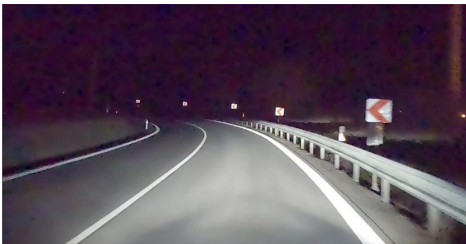
Fig. 7. An example of a well-marked curve with traffic signs [9]
