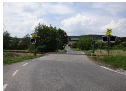
Fig. 4. - Example of adverse combination of parameters (glare, vertical curvature of the road, layout of the road).
