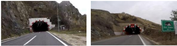
Fig. 4. Entrance in tunnel
